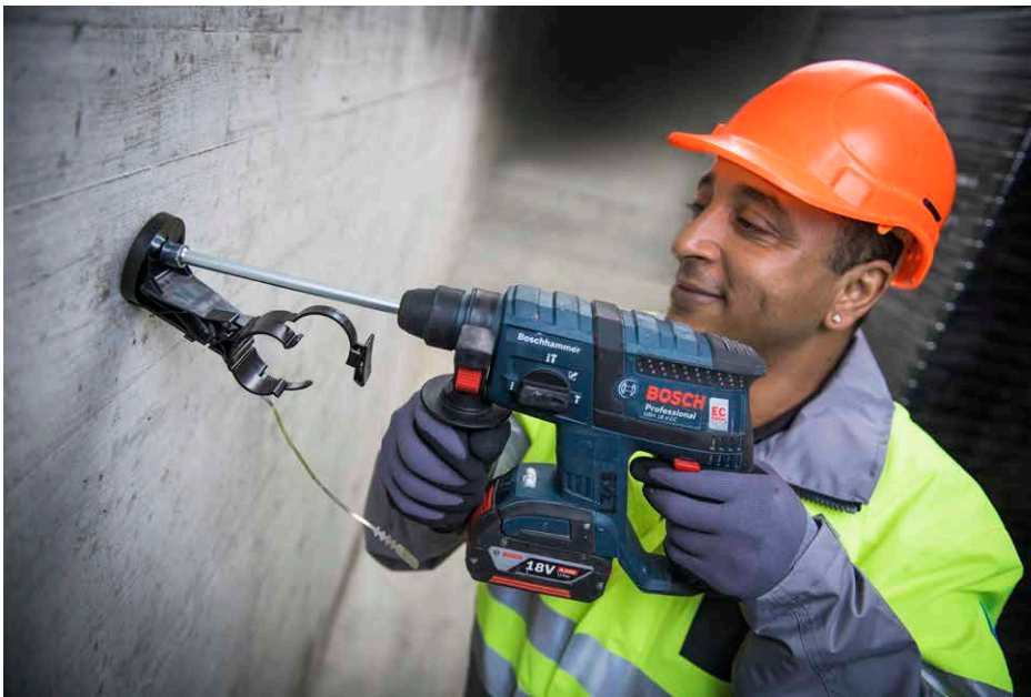
Mounting the CLIC SKH directly on the tunnel wall.
